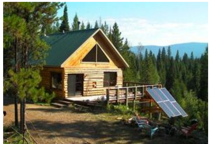
Off grid cabin well pumping
